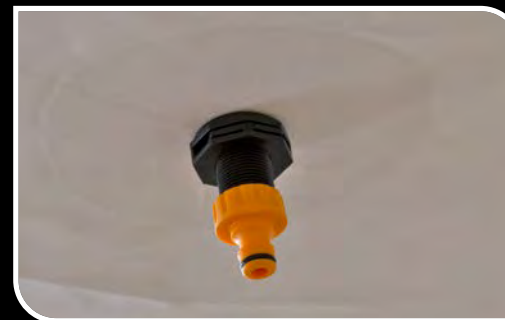
Central Drainage Point
